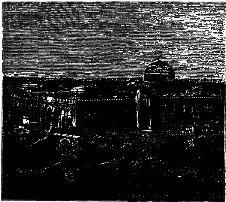
316. View of the Mosque at Kalburgah. (From a Photograph.)
